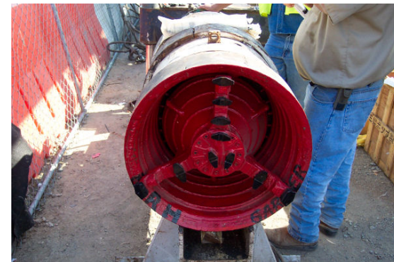
Micro TBM (Micro Tunneling)
