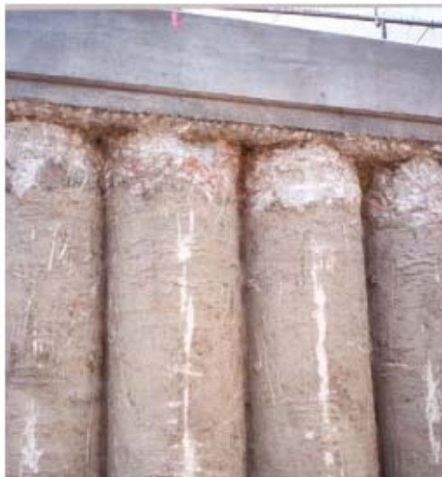
Tangent Pile Wall Construction Schematic
