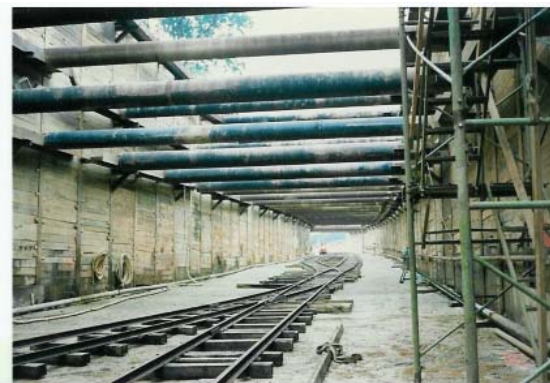
Braced Soldier Pile and Lagging Wall
