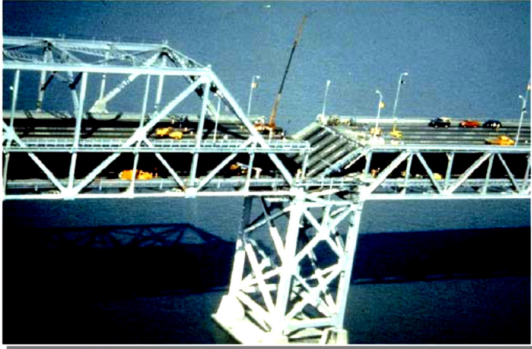
1989 Earthquake in Loma Prieta, California Oakland Bay Bridge failure.
